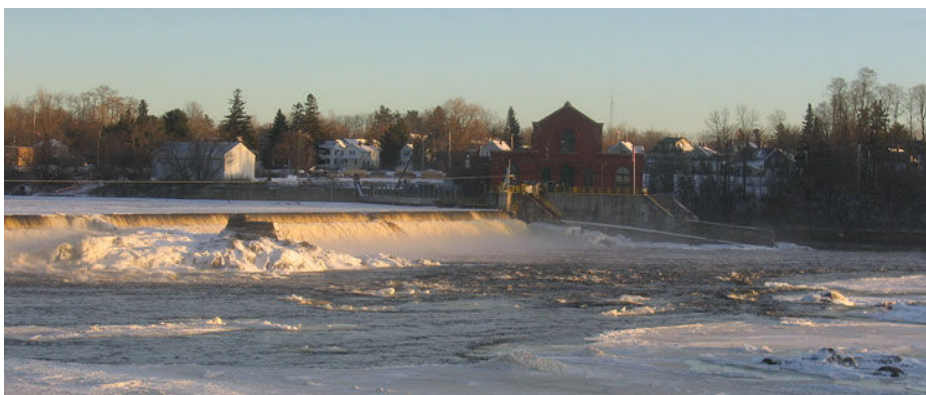
Facilities for eel passage and a fish ladder will be constructed on the Milford Dam in Old Town, Maine (Photo taken December 31, 2005).
